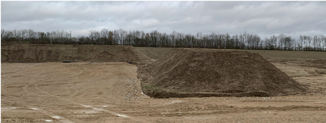
Photo 35: Topsoil Storage Example
