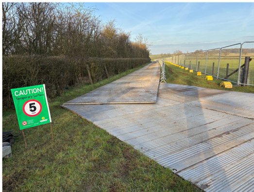
Photos 31 and 32: Removeable Temporary Trackways
